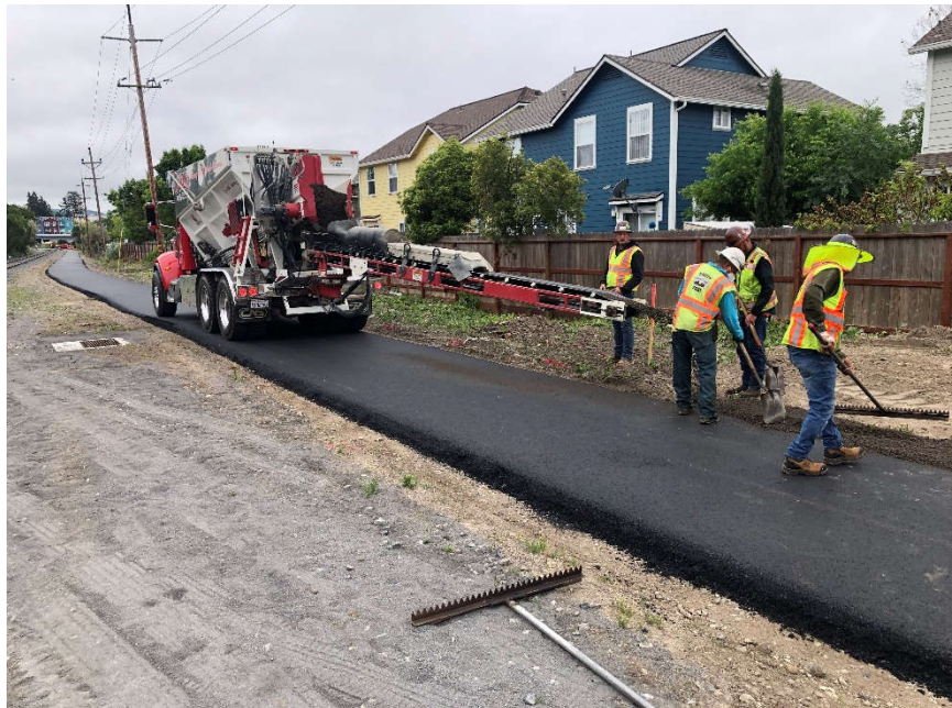
Payran to Lakeville Pathway Project
