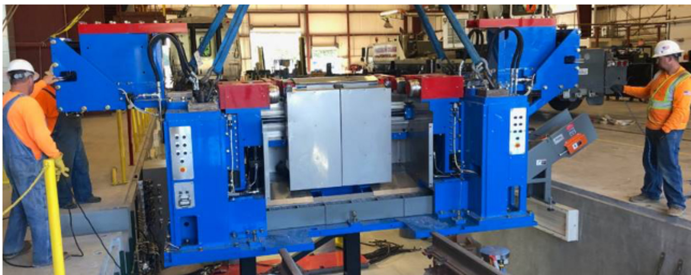
Installation of wheel truing machine
