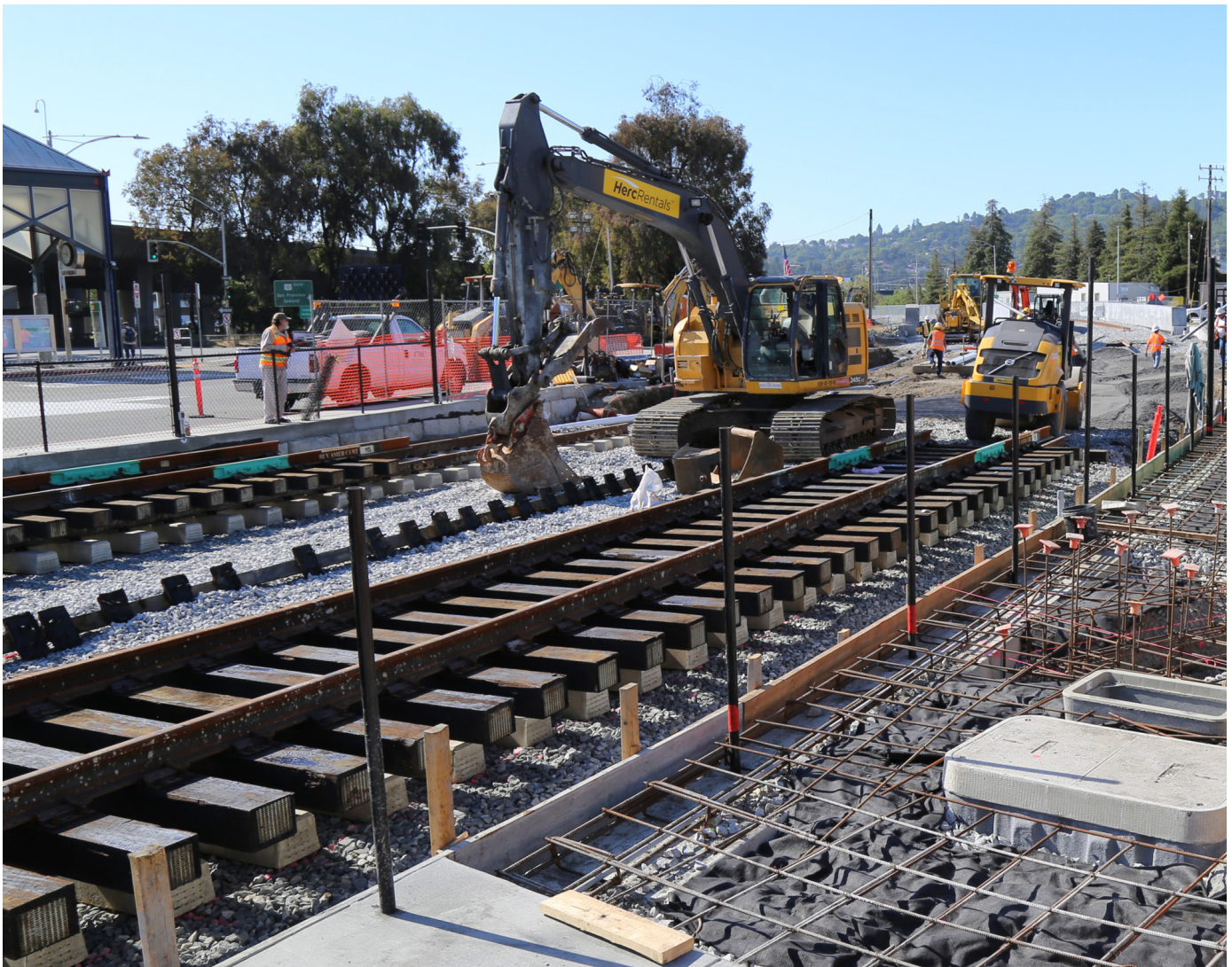
Larkspur Extension, work in Downtown San Rafael
