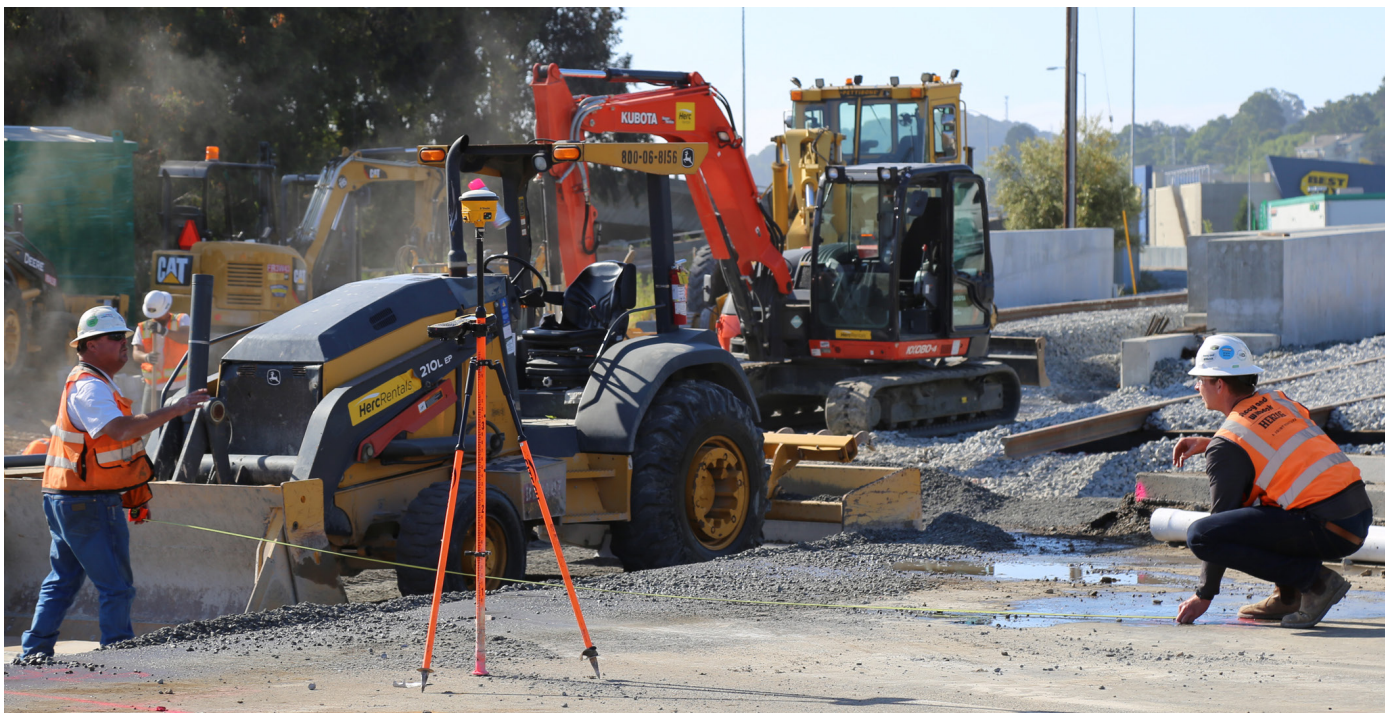
Larkspur Extension, work in Downtown San Rafael
