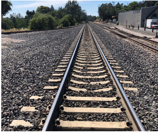
EXAMPLE OF NEW TRACK WITH CONCRETE TIES AND CRUSHED ROCK BALLAST
