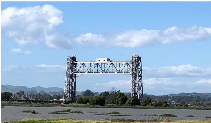
BRAZOS VERTICAL LIFT BRIDGE OVER THE NAPA RIVER
