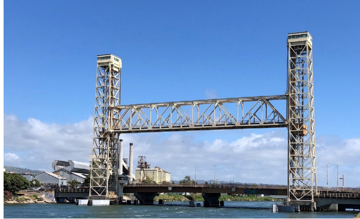
ALAMEDA-FRUITVALE RAILROAD BRIDGE
