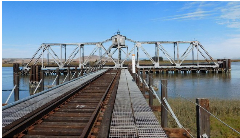
BLACK POINT SWING BRIDGE OVER PETALUMA RIVER – “OPENED” POSITION FOR MARINE TRAFFIC
