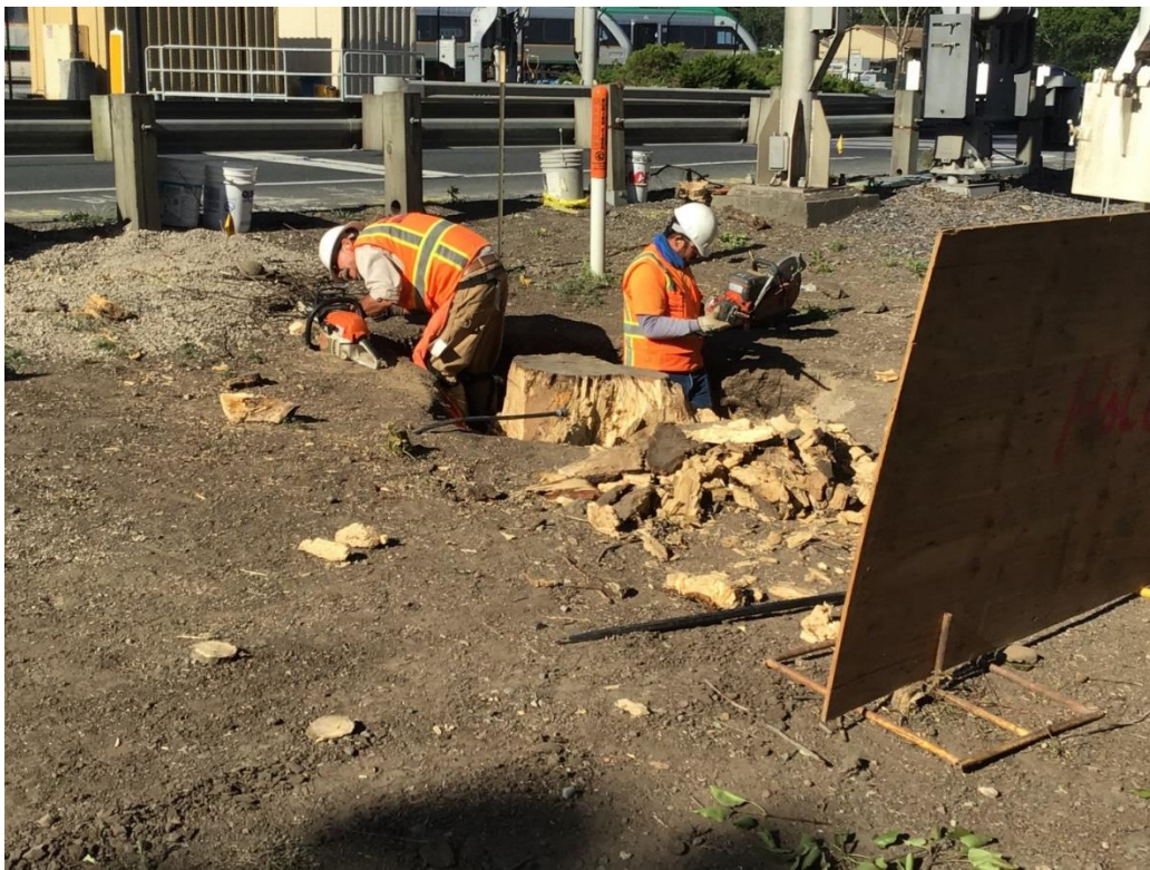
Removing a tree stump at Airport Blvd.
