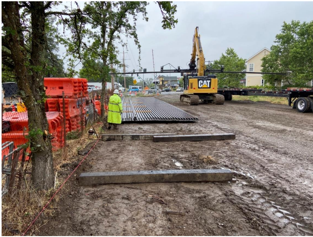
Delivery of new rail in Windsor
