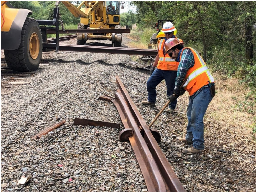
Removal of the old track south of Windsor River Road, Windsor
