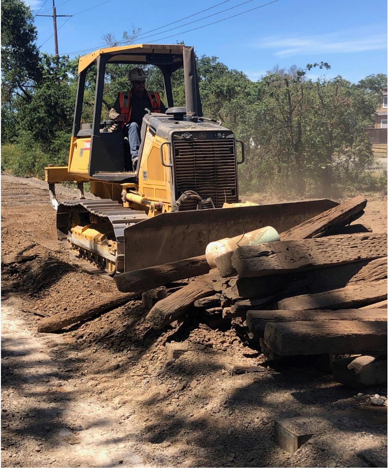
Removal of old ties
