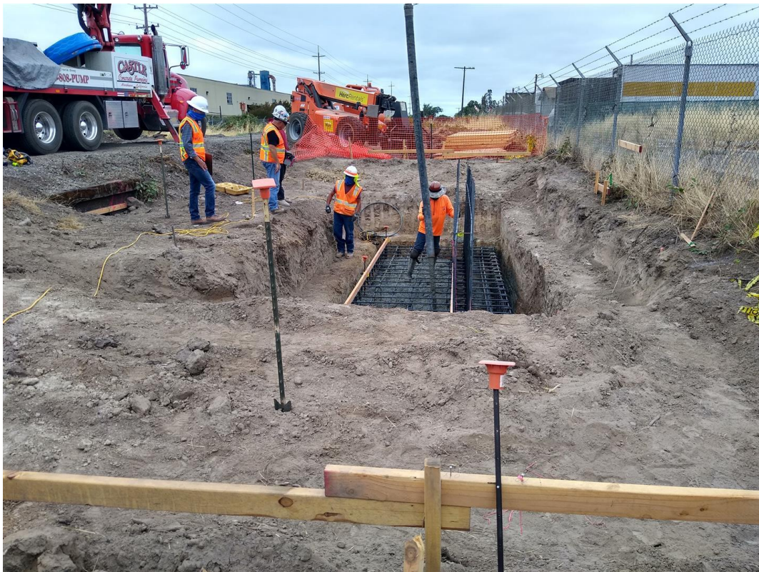
Building of Drainage Structures South of Shiloh Road
