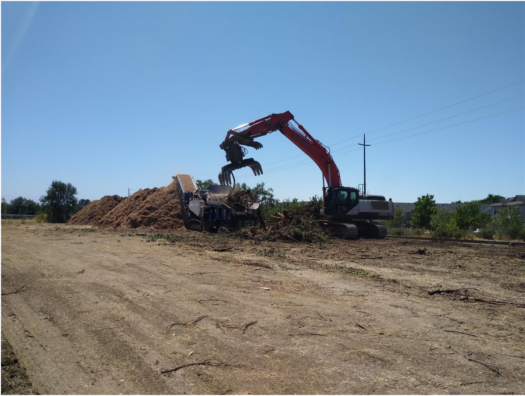
Chipping Tree Debris
