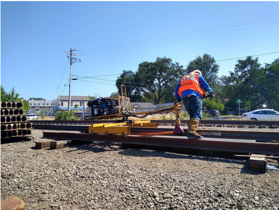
Prepping Rail for Welding
