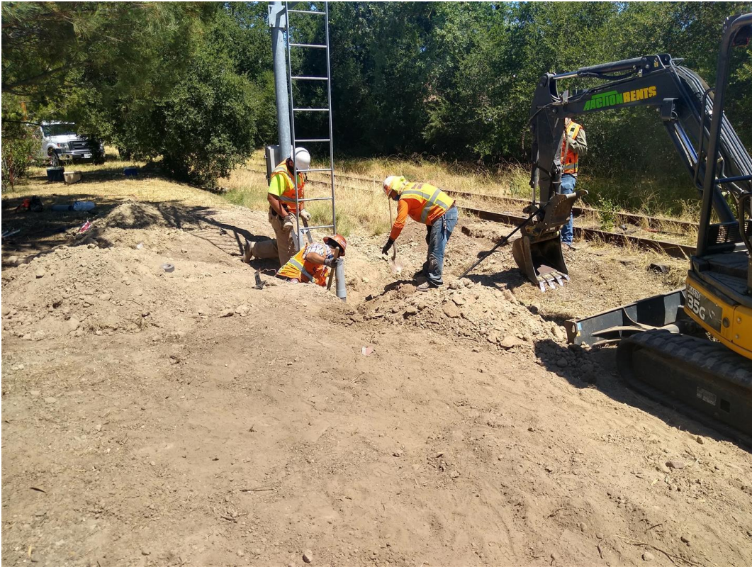
Installing Signal North of Starr Road
