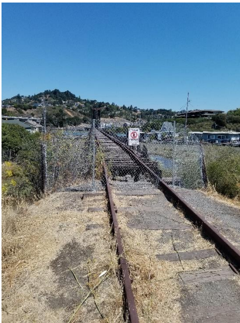
Fencing along SMART's Right-of-Way
