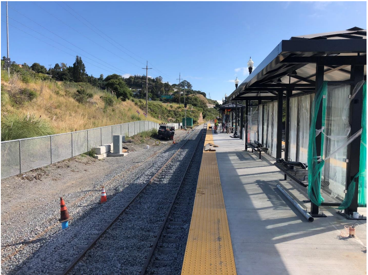
Larkspur Station Construction
