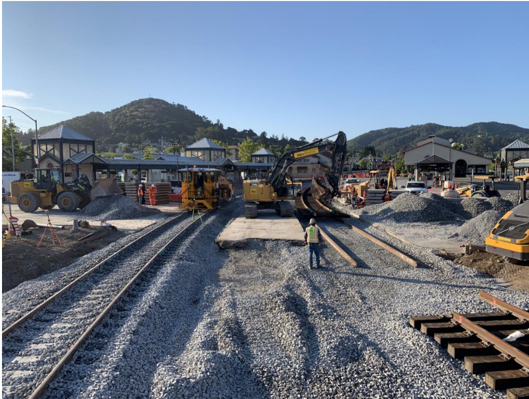
2 nd Street Grade Crossing – Track Work
