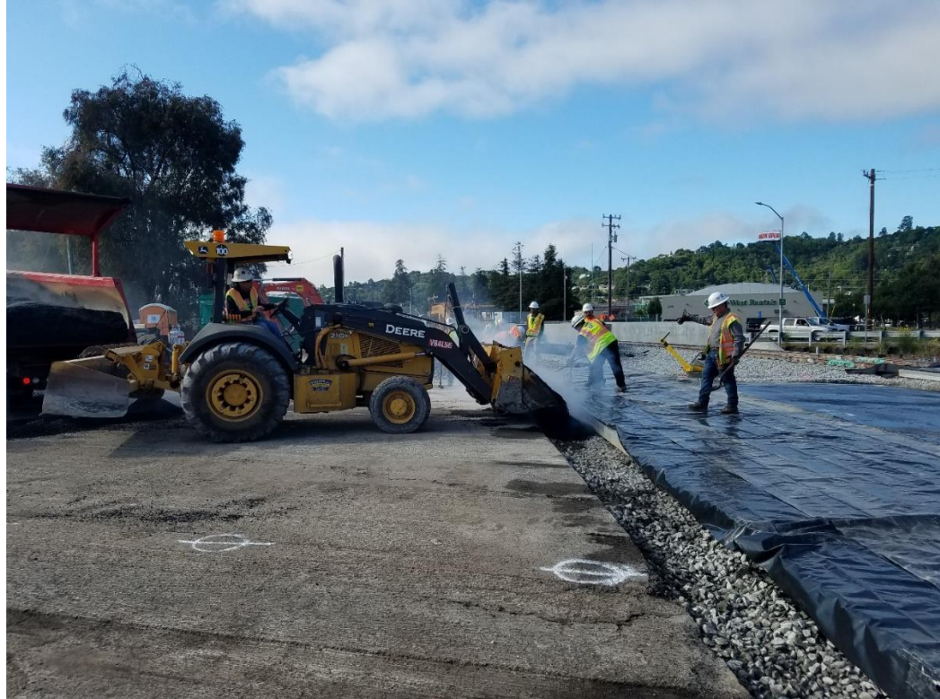
2 nd Street Grade Crossing Construction – Street Paving
