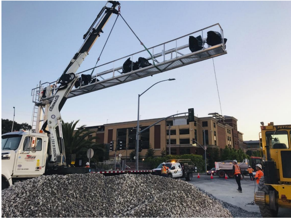
2 nd Street Grade Crossing Construction – Installation of cantilever signal
