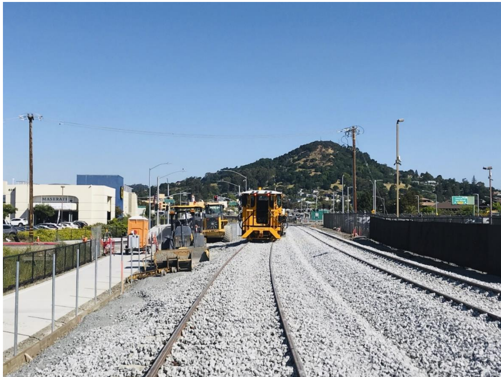
Track construction from Andersen Drive to Francisco Boulevard
