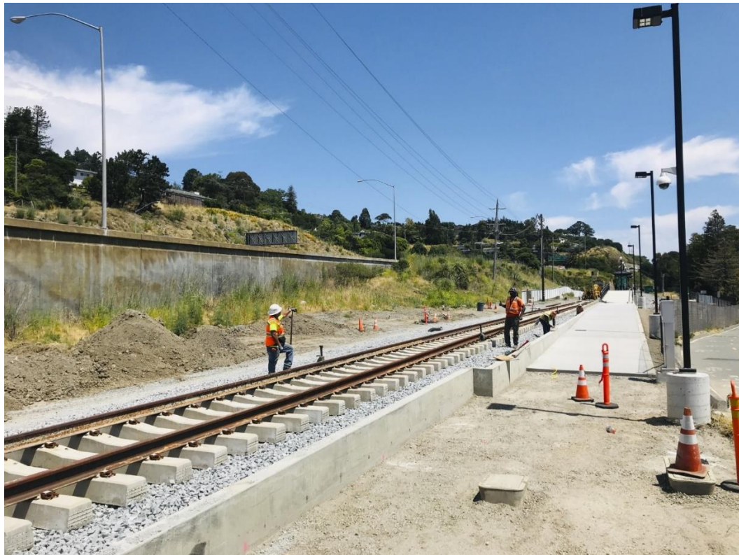
Larkspur Station – Track Construction
