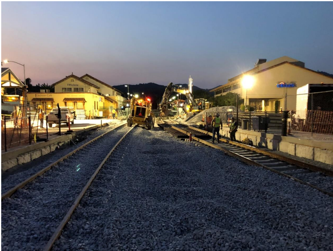
3 rd Street Grade Crossing- Track Construction (night)
