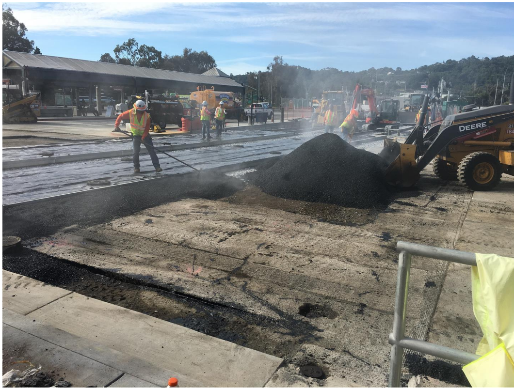
3 rd Street Grade Crossing Construction – Street Paving
